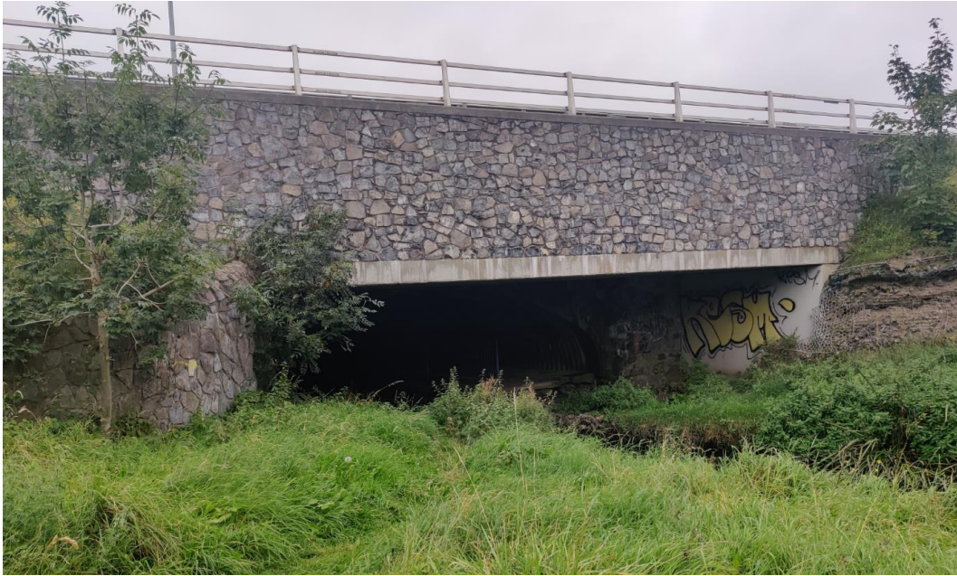
Figure 3: Existing Bridge (Southern Elevation)
